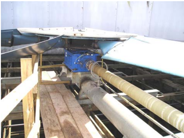
Cooling Tower Shaft Driven Gear Box
